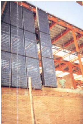
Figure 1: Intelligent building design and construction process - Mounting and integration of solar modules into the Mataró library building in Barcelona, Spain. The photovoltaic modules are at the same time façade elements and are part of the solar power station (53 kWp). Source: tfm, Spain.
