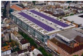
Figure 5: Architecture and marketing - PV installation of 240 kWp mounted on the Convention Center Basel, Switzerland. Solar electricity is marketed within the local solar stock exchange. Source: photo from Convention Center Basel, montage picture from energiebuero® Zurich, Switzerland
